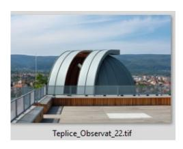
Conical titanium zinc shares for the domes and the elegant curve of the opening wings provide a functional, but also visually exciting architecture. A special challenge was the (impact-)rainproof connection of the movable wings to the rotating dome.
